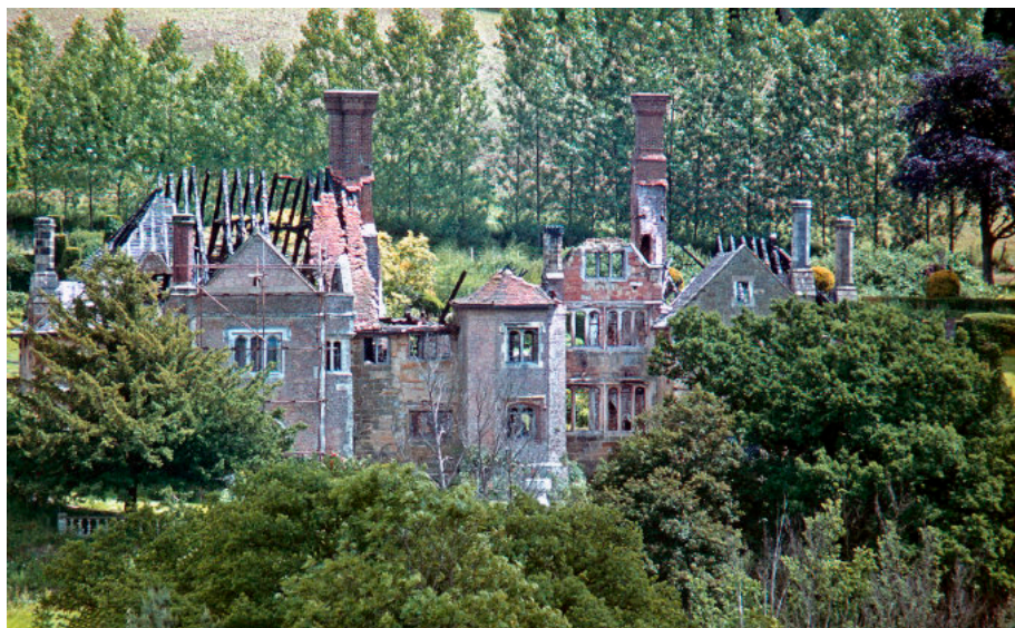
Brede Place in June 1980 awaiting repair. John Crook
