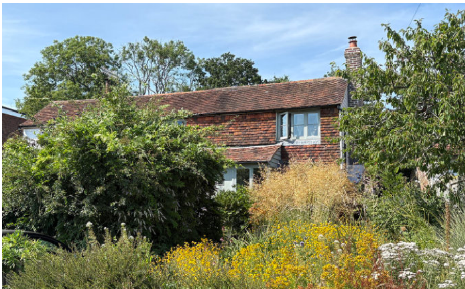
Seymour Cottage (centre), one of a group of three cottages.
