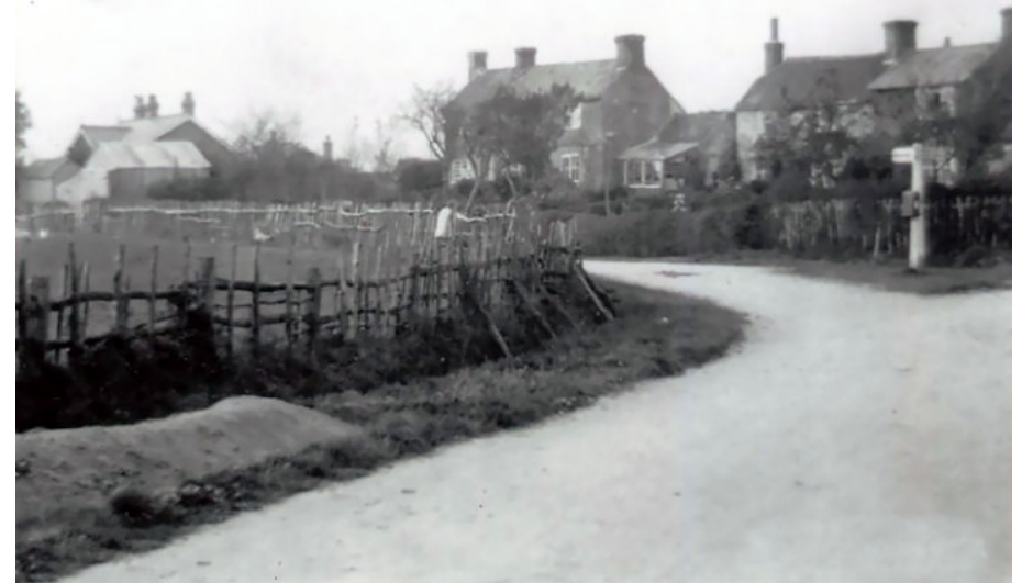
View north up the A28 and the junction with Pottery Lane, 1920s.
