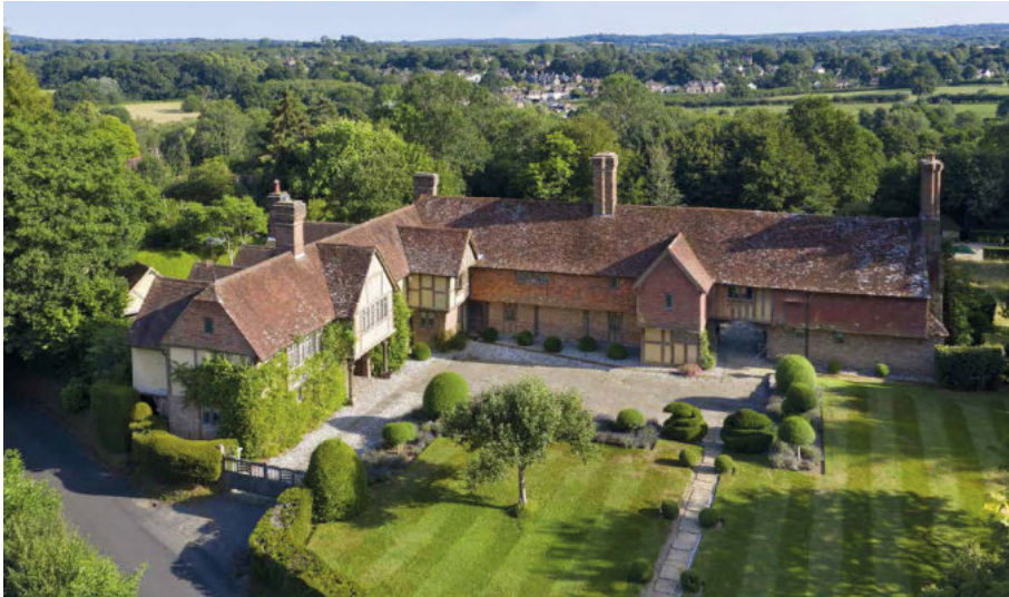
Court Lodge rebuilt at Groombridge.
